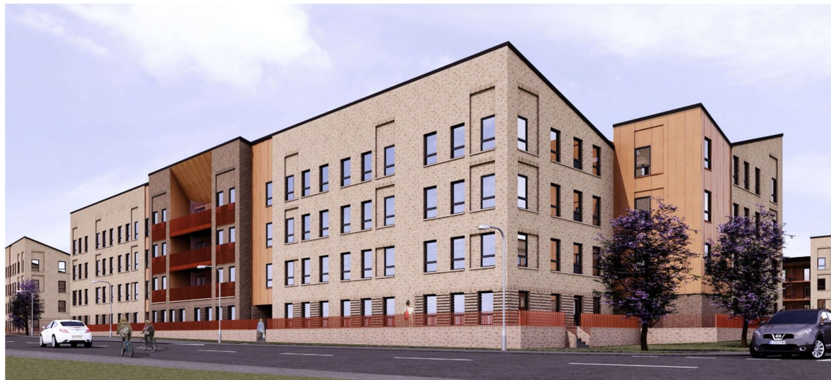
Ashleigh Construction – Butterbiggin Road, Glasgow
